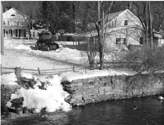
Retaining wall collapse near Shaker Mill Dam. Photo by Doane Perry.
