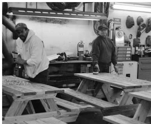
John Lyford and Thom Lipiczky (right) building picnic tables at the Highway Department garage. Photo by Bob Salerno
