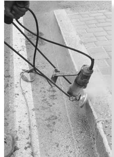
Highway Department worker grinds curb to reduce damage to tires. Photo by Curt Wilton.
