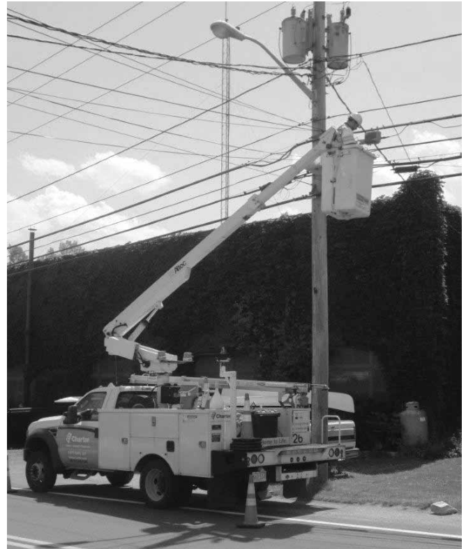
Charter (now Spectrum) technicians have been busy rewiring and upgrading equipment around town. Photo by John Parker.
