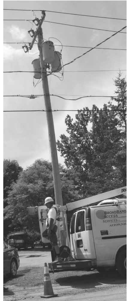
This utility pole carries power, transformers, cable TV, and telephone service. Photo by Doane Perry.
