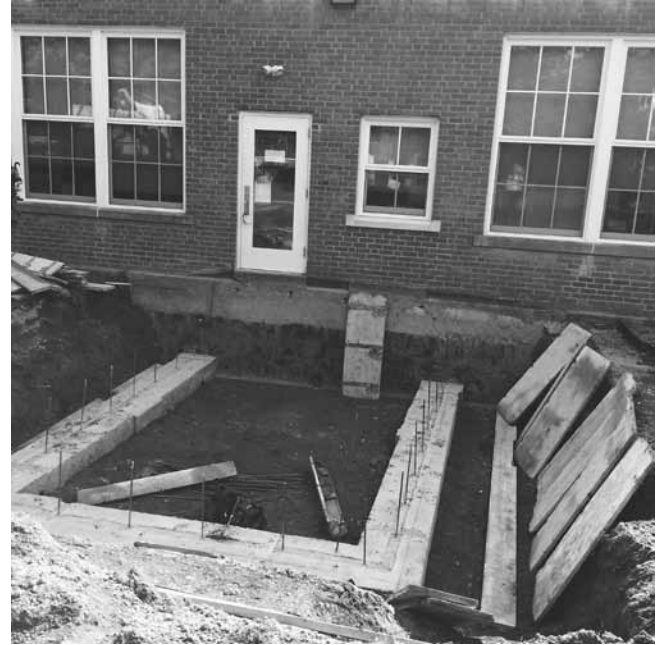
Coming soon: new library entrance under construction. Photo by Lee Appelbaum.
