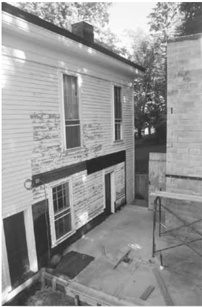
This new structure behind the Old Town Hall will house the elevator, three bathrooms, and additional access. Photo by Bob Salerno
