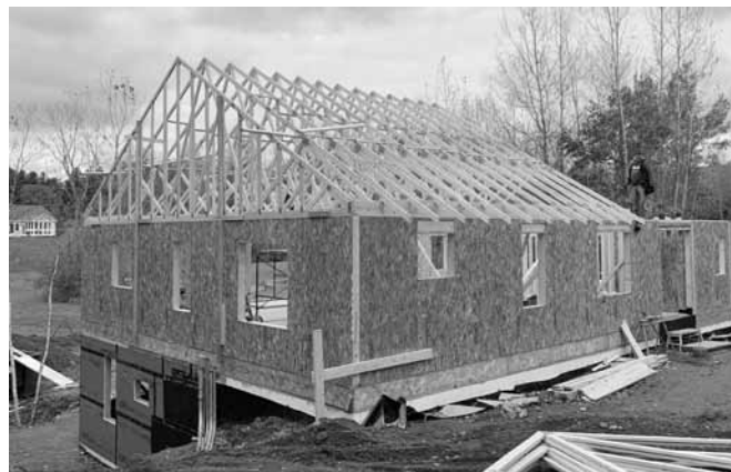
The house began to take shape after a huge crane lifted the trusses into place. Photo by Mike Wilser
