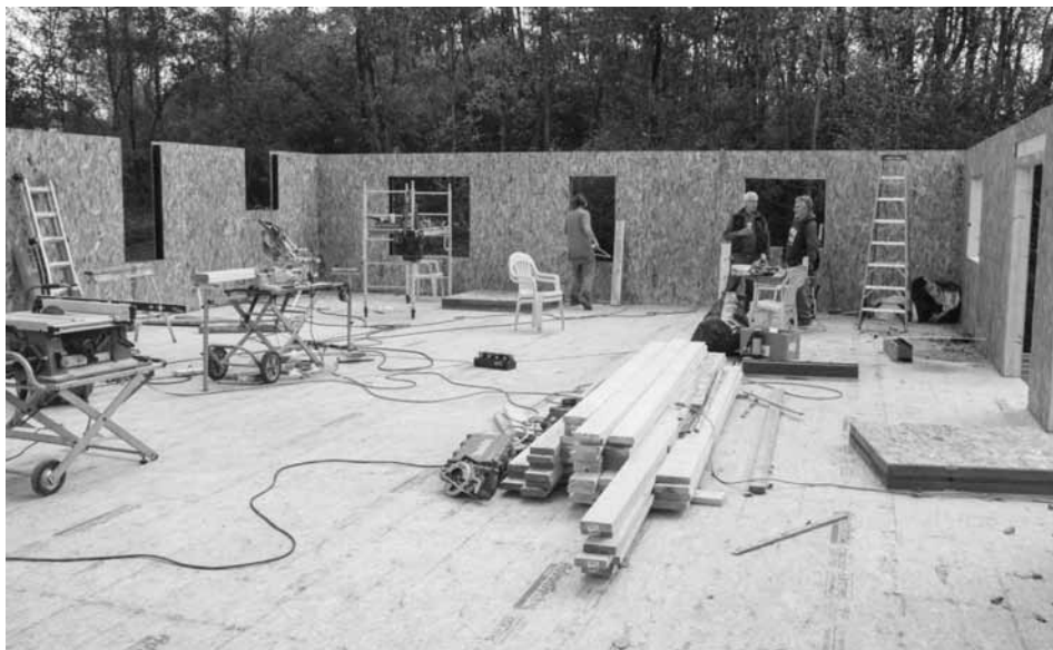
Interior view of SIPs on the main floor with some of the window and door openings cut out. Photo by Mike Wilser
