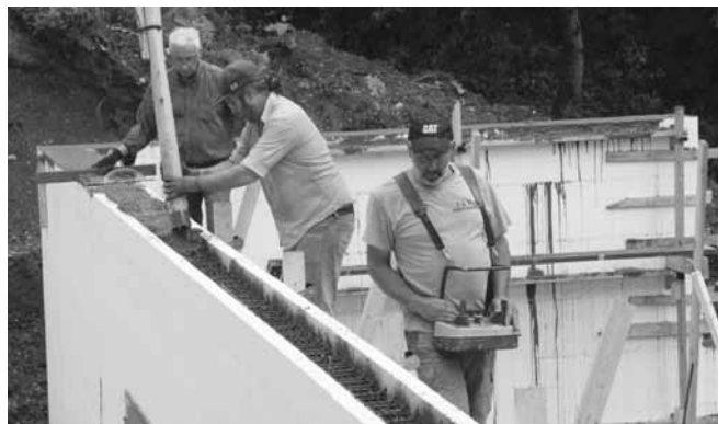
Thom, Arthur, and Jeff, the concrete pump operator, pouring the wall. Photo by Mike Wilser
