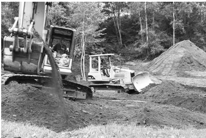
Excavation begins at the new house site. Photo by Thom Lipiczky
