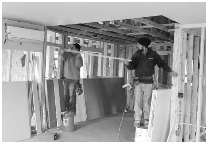
Two workers from the Bierbower Drywall & Plaster Company create a ceiling, so insulation can be blown in above. Photo by Thom Lipiczky
