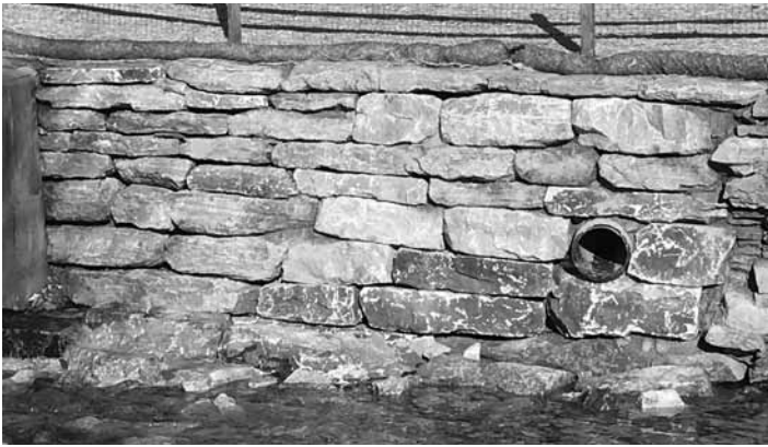
Contractor Dennis Lamke repaired the collapsed Williams River wall and drain pipe. Photos by Doane Perry
