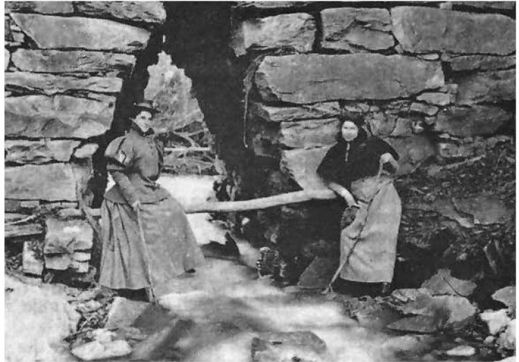
Bailey Brook Bridge. Image courtesy of West Stockbridge Historical Society
