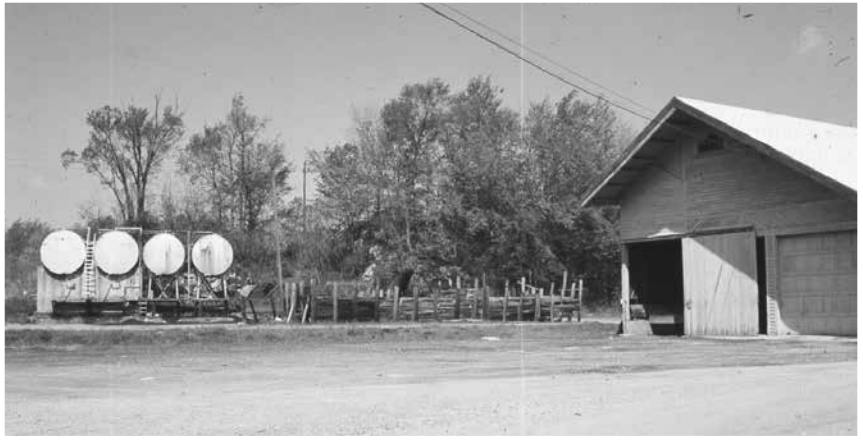
Depot Street Tanks. Photo courtesy of West Stockbridge Historical Society
