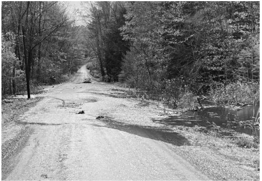
Flooding, West Alford Road
